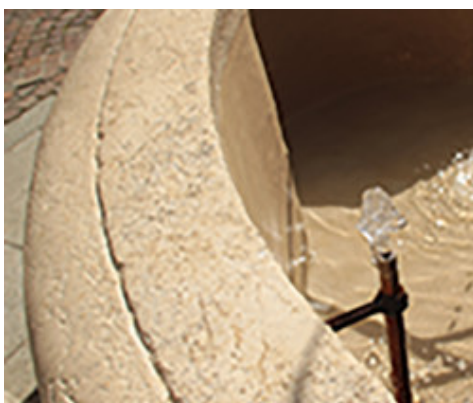
Waterproofing the basin of a stone fountain
