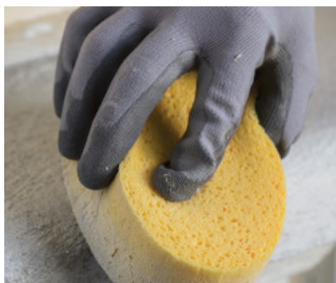
Finishing off Mape-Antique Ecolastic with a sponge float
