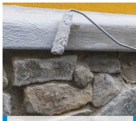
Waterproofing a wall cap with Mape-Antique Ecolastic
