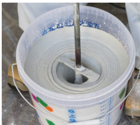
Mixing Mape-Antique Ecolastic
